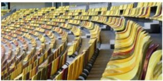
The seat is made of polyamide or polypropylene – materials that have excellent mechanical and physicochemical properties – and its supporting structure is made of corrosion-proof steel. The durability is increased by its strengthened edges.
